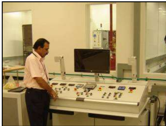
Control Desk under Installation
